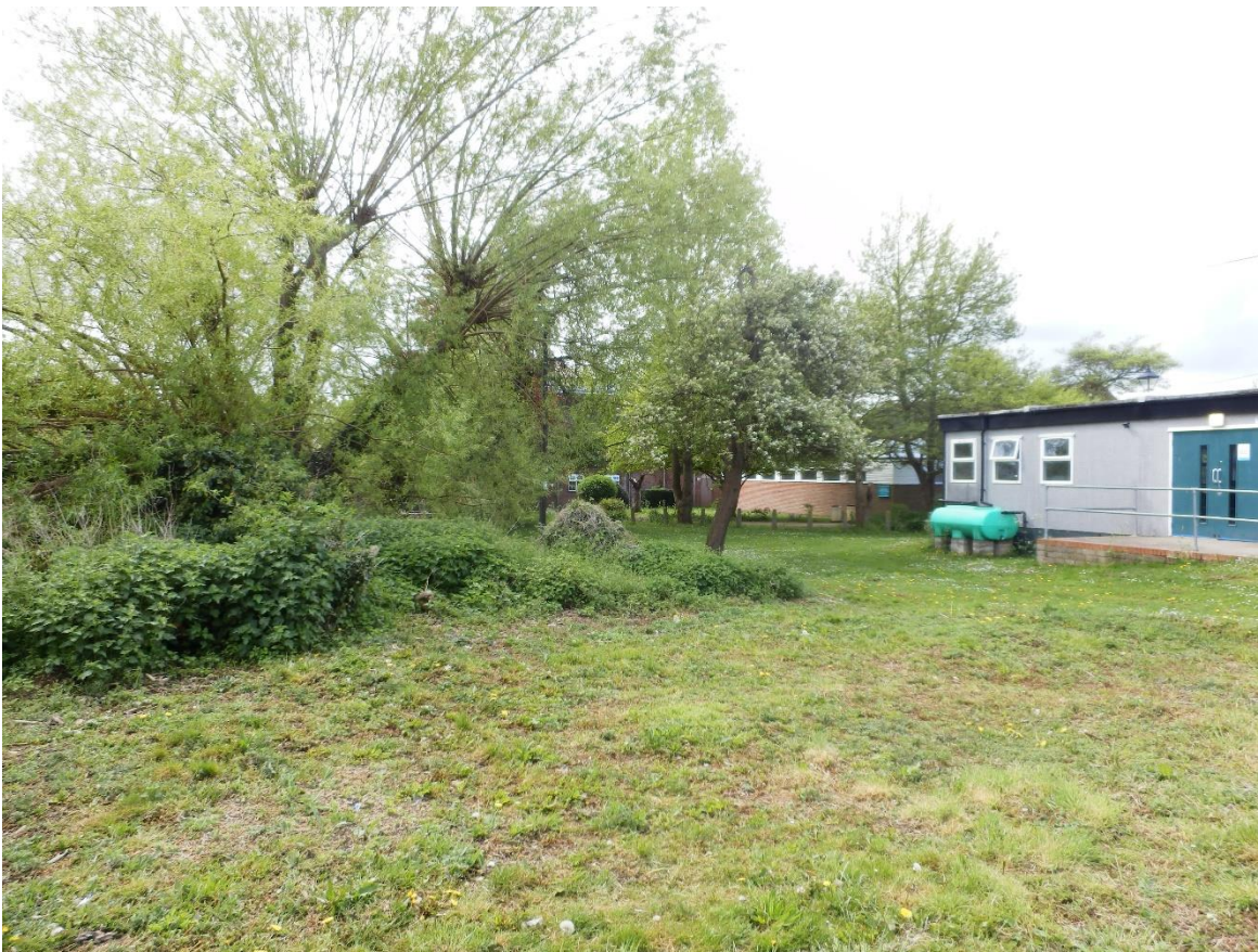
Existing Greenhill building (eastern side looking south)
