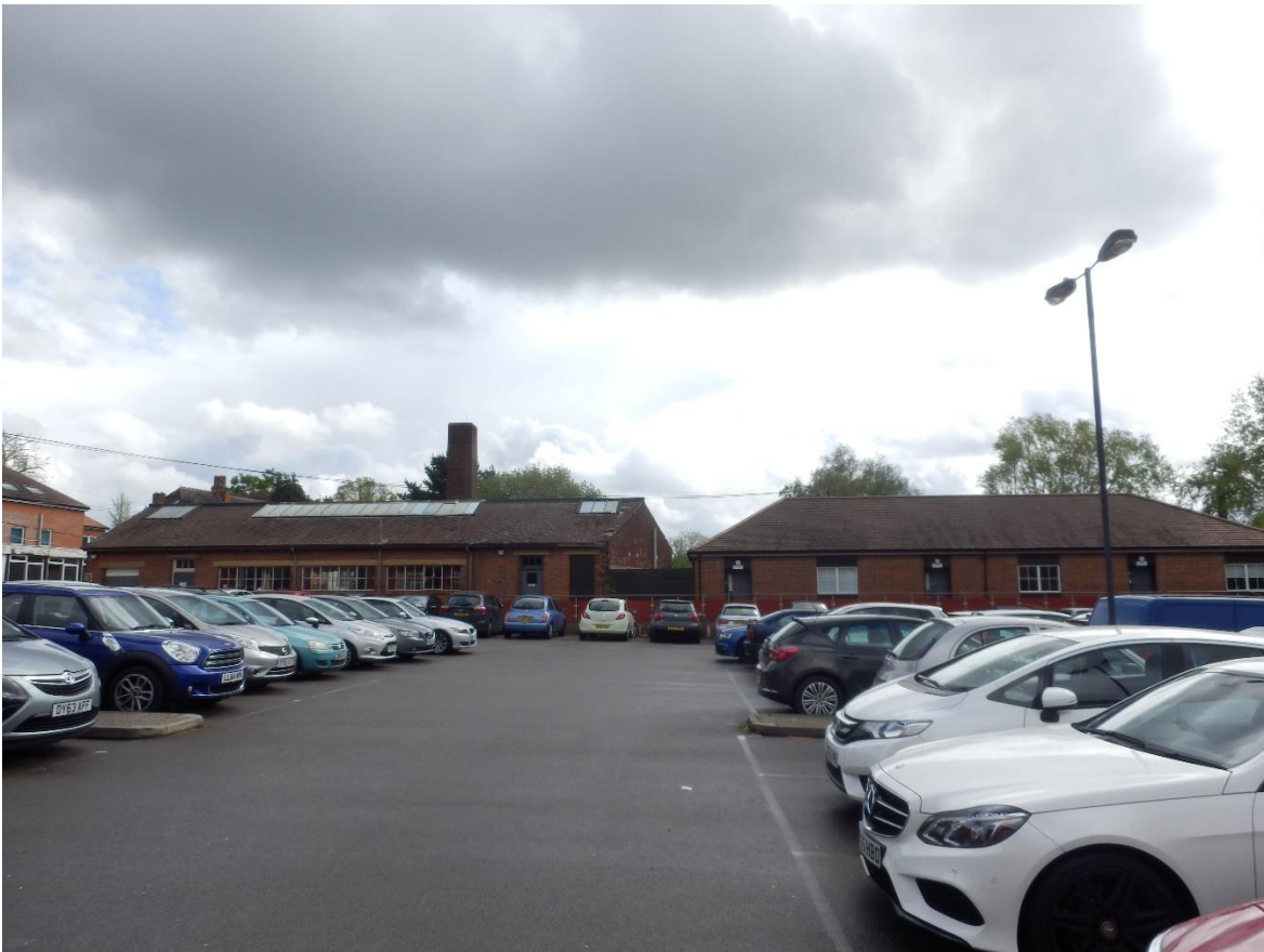
Car parking looking toward buildings adjacent to the site (Grimsdyke, Hatch End)
