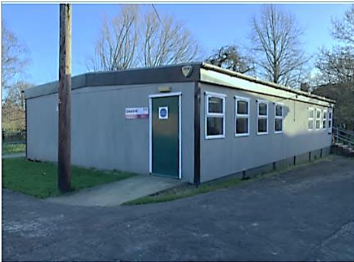
Existing Greenhill building (north side)
