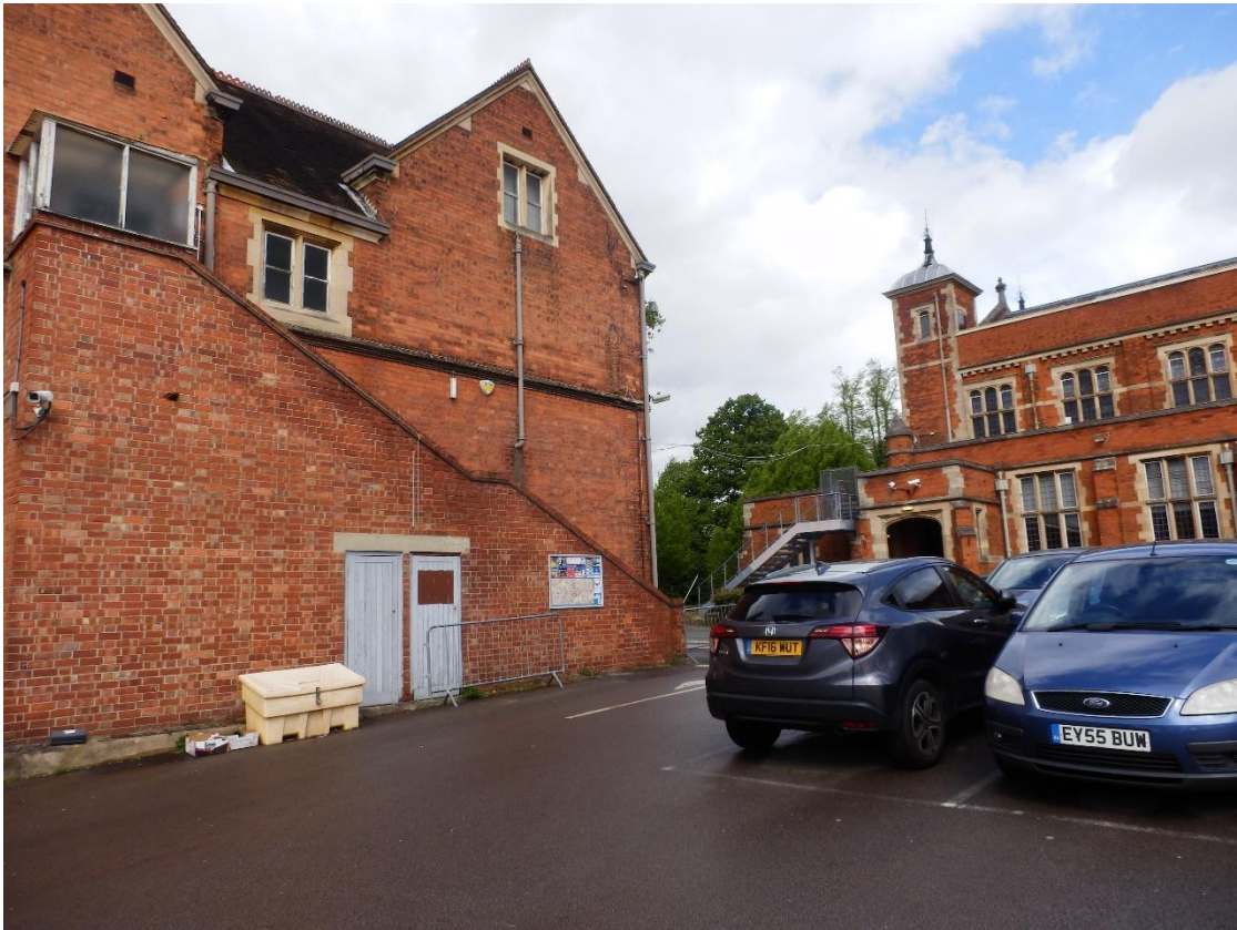
Car park showing part of rear of Elliot Hall and the Art Block (locally listed)
