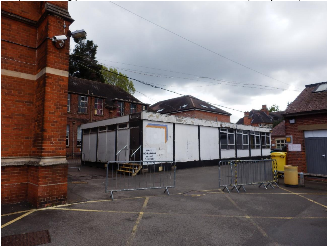
Portacabin to be demolished
